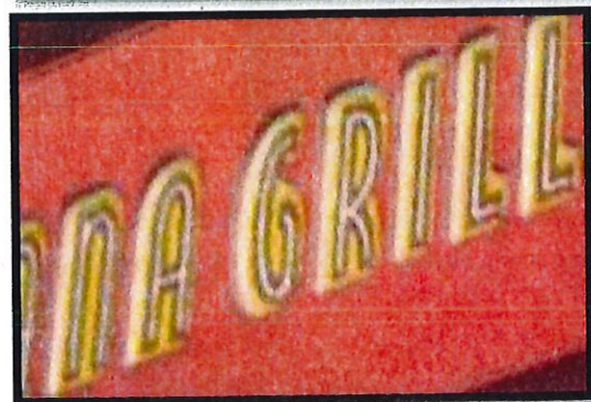
Push-thru or routed out letters and graphics are encouraged to provide dimension
