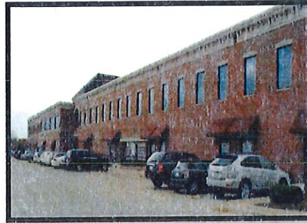
(CORNICES) Public entrance in rear shows architectural details
