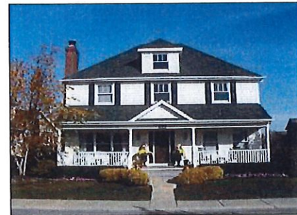
Adding outdoor space for residents to relax and interact with neighbors, porches may extend along part (top) or the entire length (bottom) of the front elevation. Also, the dormer shown in the bottom image displays architectural style and proportion consistent with the rest of the home.
