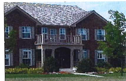
In addition to the dual gables, the roofline of this home is enhanced using eaves that subtly overhang the front façade.
