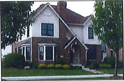
Brick or stone shall be used on a chimney when it is located on a front elevation (shown to the left) or side elevation facing a street.
