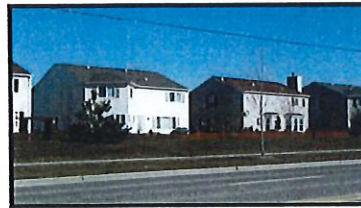
The single family homes shown above are through lots as defined by two distinguishing features: the visibility of the rear elevations from an exterior neighborhood street (foreground) and visibility of the front elevations from an interior neighborhood street (not shown).
