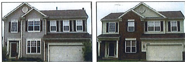
Both images illustrate the use of trim around windows to enhance the exterior architecture of the homes. The image on the left illustrates the use of similar ornamental trim around the doorway and windows to create a uniform building design. The image on the right illustrates how window trim can be incorporated on a brick elevation.
