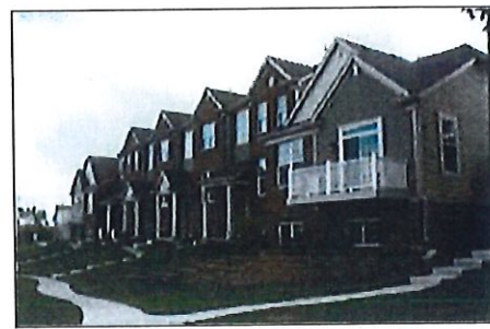
Brick is one of the preferred building materials for residential homes in the community. Homes may incorporate a single material (above) or a combination of materials (below).
