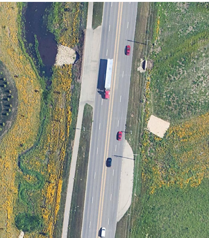
Figure 18. Truck Pullouts in Kane County, IL
