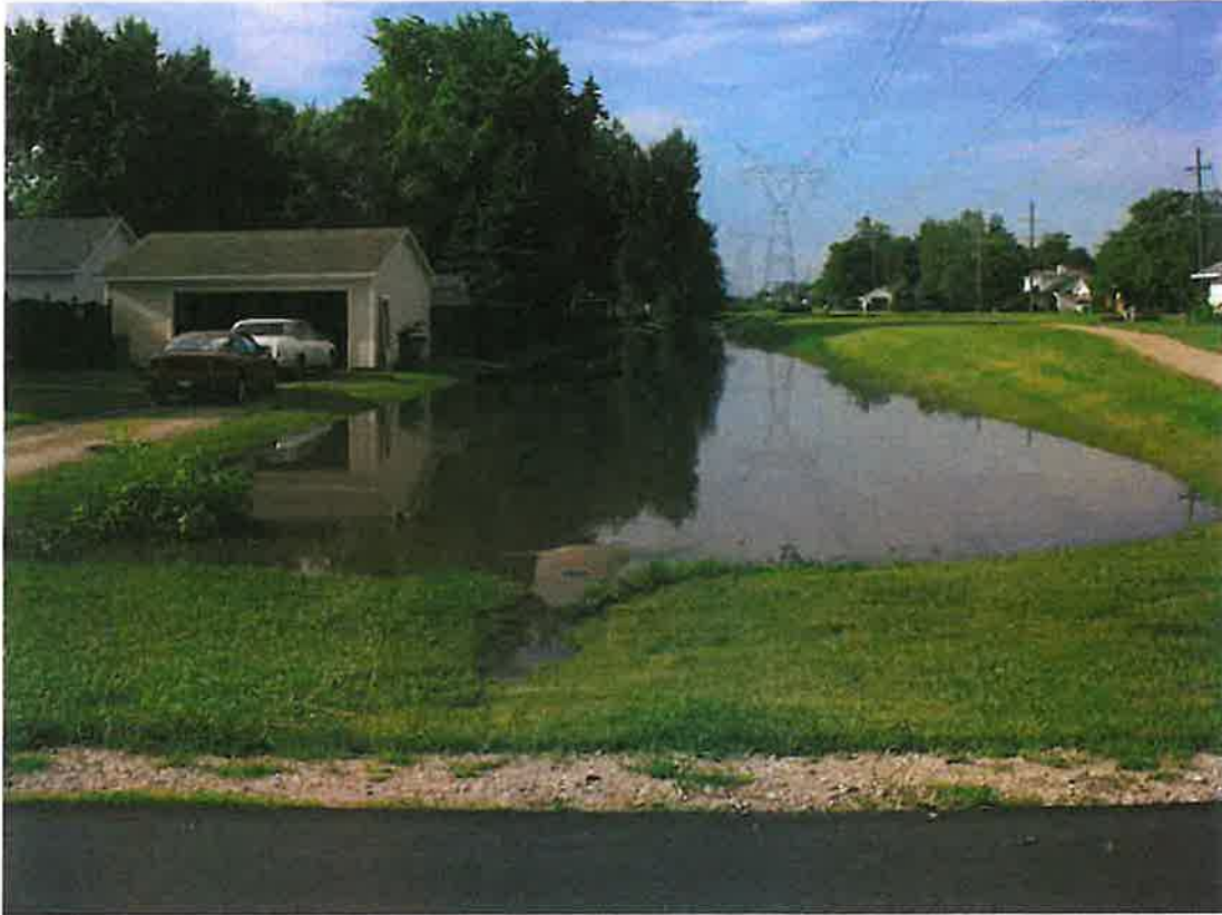
Condition of “ComEd” ditch a day after rainfall event – Oak Street looking south, 6/22/09
